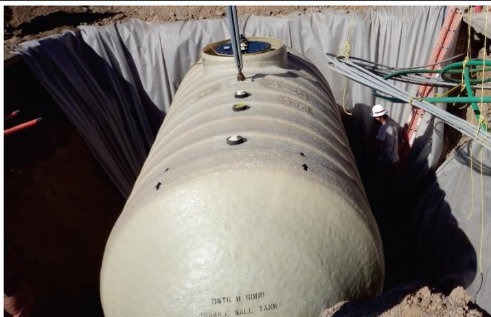
**Figure 6-1** Underground storage tank (note worker at right for scale). Courtesy of NMED Petroleum Storage Tank Bureau.
